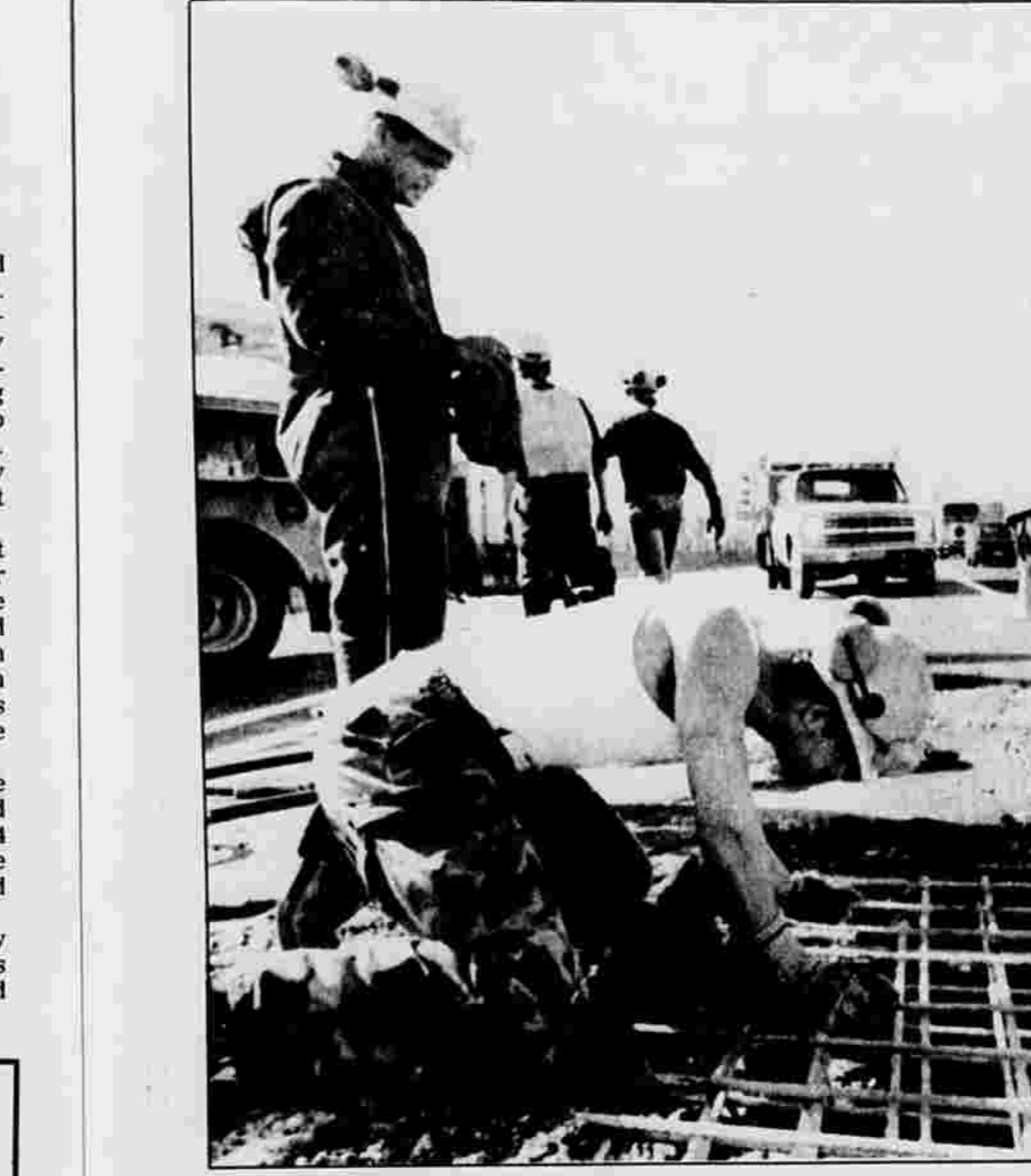
LOOKING DOWN — James Harris, a state worker, peers into an 18-inch hole discovered Wednesday in the deck of the Interstate 95 bridge over the Rippowam River in Stamford.
